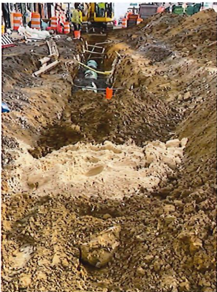
Figure 4: View of 21" SDR Sewer Main installation
