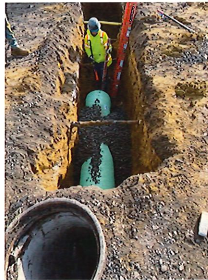
Figure 5: View of 21" SDR Sewer Main installation
