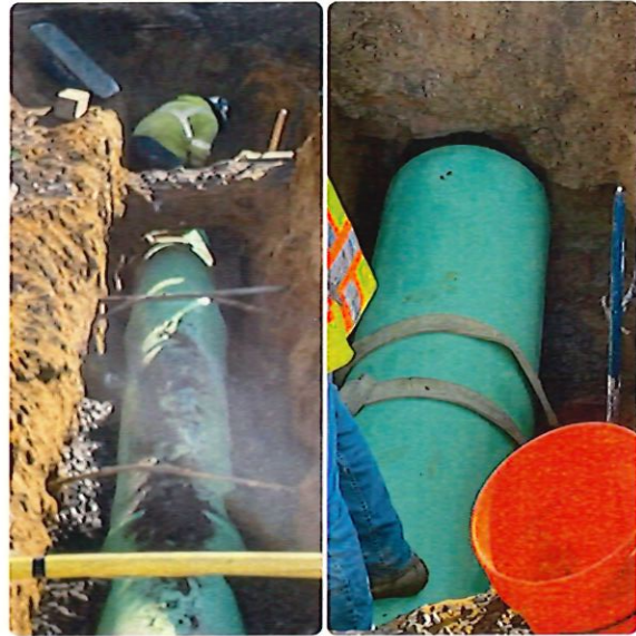
Figure 3: View of 21" SDR Sewer Main installation
