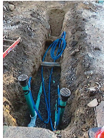
Figure 5: View of sanitary service connection installation /future water service connection
