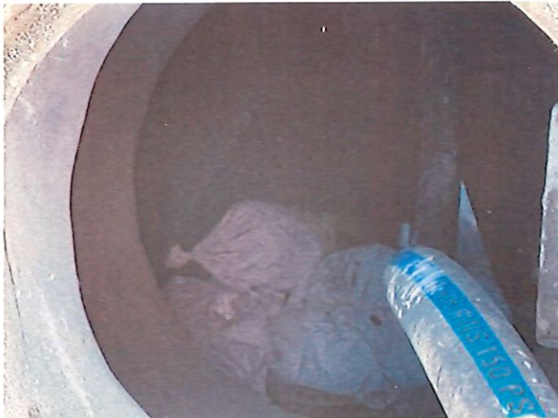
Figure 4: View of manhole sandbagged for bypass pumping
