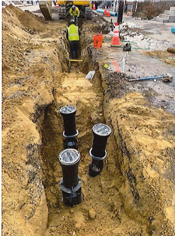
Figure 1: Backfilling of services
