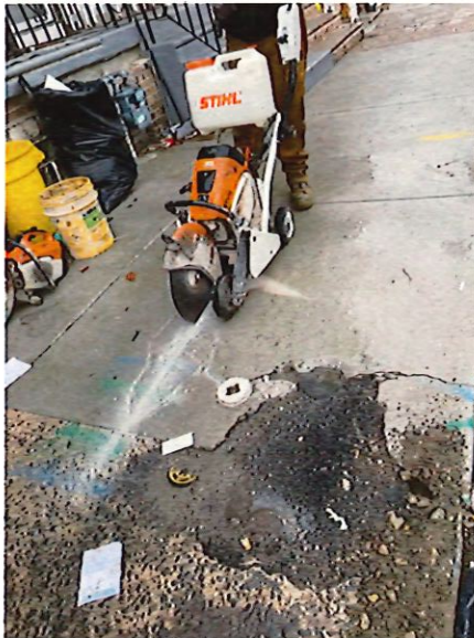
Figure 4: Preparation of service connections
