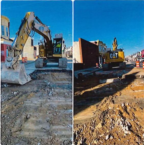
Figure 2: View of pavement removal
