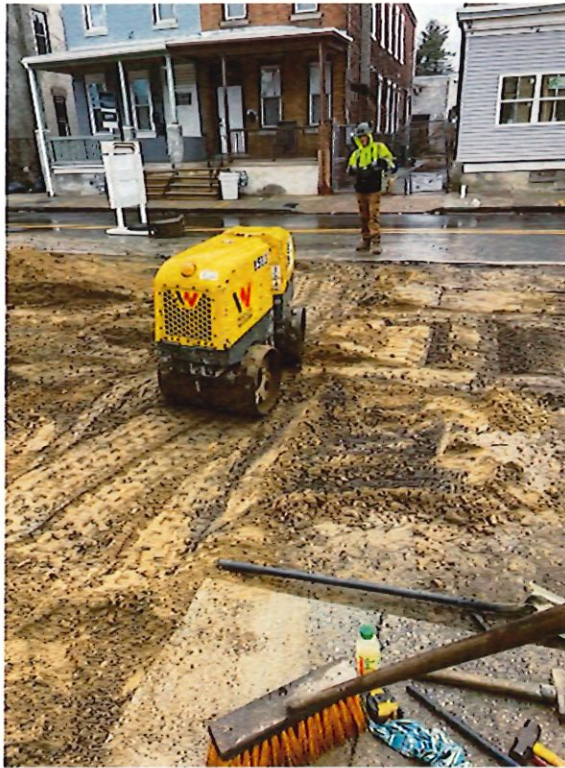
Figure 1: View of trench being compacted
