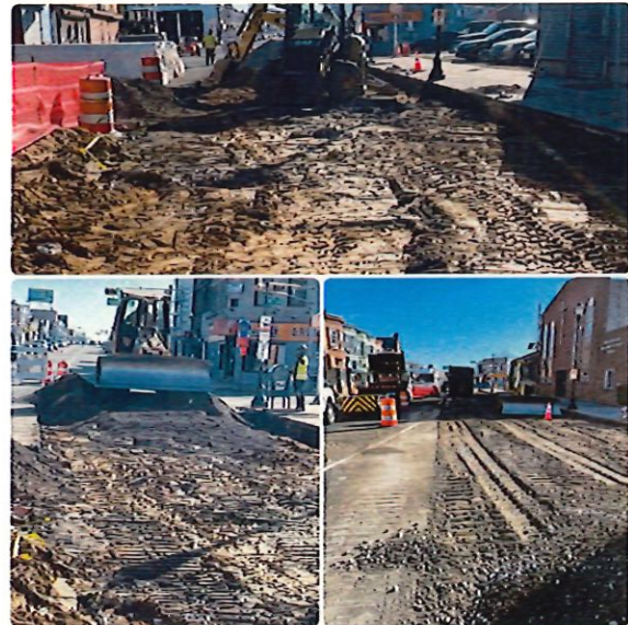
Figure 5: View of pavement removal
