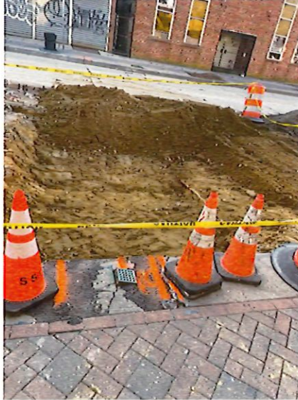
Figure 2: View of test pit being performed to verify utility conflict
