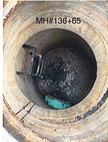
Figure 3: View of manhole after power washing
