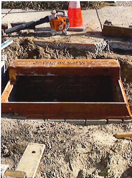
Figure 4: View of reconstructed type B Inlet
