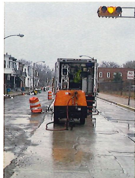
Figure 5: Videoping pipe inspection being performed
