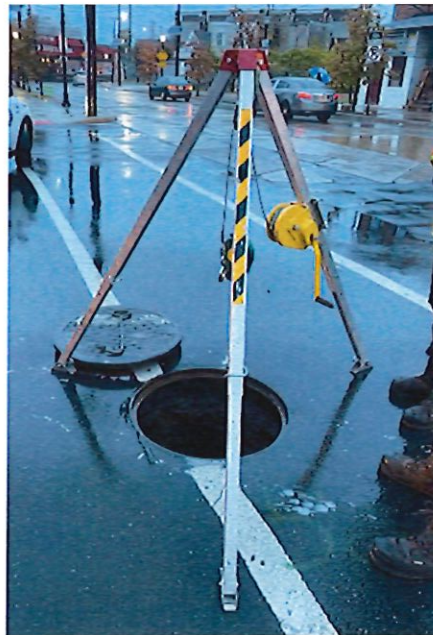
Figure 1: View of safety retrieval system set up for use
