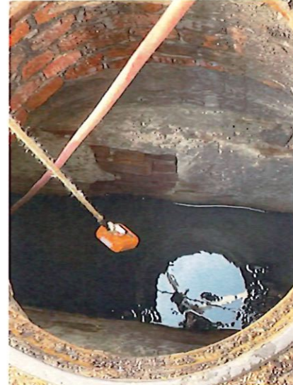
Figure 3: View of manhole being air tested
