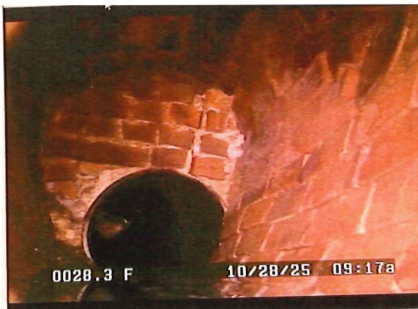
Figure 4: View of cleaned existing pipe
