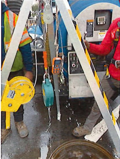
Figure 2: View of tri-pod being setup
