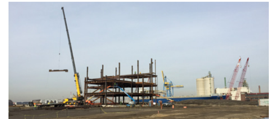
^ SITE OF THE FUTURE WORLD HEADQUARTERS FOR HOLTEC INTERNATIONAL
