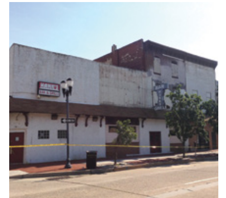
MARKET STREET FACADE IMPROVEMENTS BEFORE (TOP) AND AFTER (BOTTOM)
